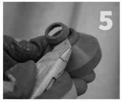
Cut the EPDM collar to appropriate conduit size (see Drawing 1, Detail B on cover).
