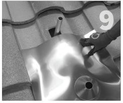
Bend the flashing to follow the contour of the tiles. Place flashing over conduit and tuck it up under the next course of tiles.
