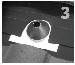
Clear away any dust and debris and install subflashing. Waterproof at underlayment level according to roofing manufacturer instructions and Tile Roofing Institute Guidelines.
