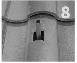
With a diamond blade on a grinder or skill-saw, cut tile to allow conduit to pass through. Place cut tile back in position.
