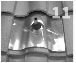
rubber to both the flashing and the conduit in the all the way down to the flashing. location of the EPDM collars final position.
