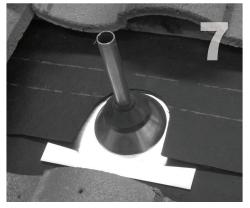
Slide the collar over the conduit all the way down to the flashing.
