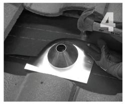
Under the top layer of felt, secure the subflashing with 2 roofing nails at the top corner of the subflashing. Apply sealant over the nail heads.
