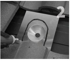
Apply sealant compatible with the roofing material on the underside of the subflashing in and upside down U.
