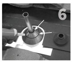
Apply a bead of sealant compatible with both the roofing material and EPDM rubber to both the flashing and the conduit in the location of the EPDM collars final position.
