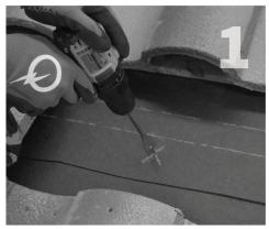
Drill your conduit hole next to the rafter so you can secure the conduit below the roof surface (see Drawing 2). For 1/2" conduit, drill a 7/8" hole; for 3/4" conduit, drill a 1" hole; for 1" conduit, drill a 1-1/4" hole.
