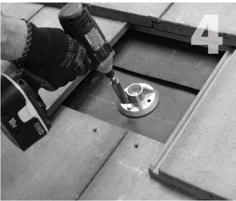
Align QBase over rafter center and drill two 7/32" pilot holes. Place grade-8 machine bolt under QBase in hex slot, threads pointing up. Lag QBase into rafter on marks.
