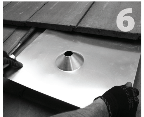
Cut a hole in the tile removed, with room to get the post through. Replace tile in position. Insert post and tighten into place. Install the 18"x 18" flashing and apply sealant around the opening.
