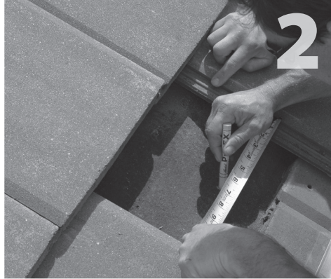
Locate and mark center of rafter.
