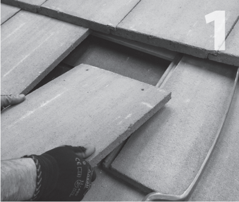
Remove tile at selected location of mount.
