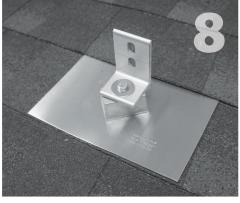
Using a 1/2 inch socket on an impact gun drive the lag screw until the QBlock stops rotating easily. **DO NOT over-torque.**
