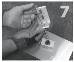
Slide the washer and the L-foot (not included) onto the lag screw.
