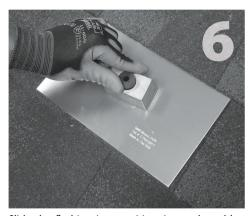
Slide the flashing into position. Insert the rubber plug into the QBlock cavity.
