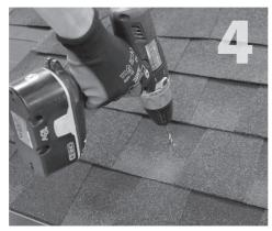
Using drill with 7/32" bit, drill pilot hole into roof and rafter, taking care to drill square to the roof. Do not use mount as a drill guide. Drill should be 'long style bit', aka 'aircraft extension bit' to drill a 13/4" deep hole into rafter.
