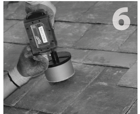
Using a 4" diameter diamond hole saw and the pilot hole drilled in step 3, drill through the existing slate.
