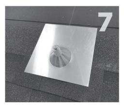
Install flashing over mount.
