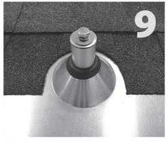
Apply sealant where post and flashing meet. Install EPDM counter flashing collar. Seal post with hardware if not installing racking right away.
