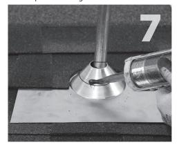
Apply a bead of sealant compatible with both the roofing material and EPDM rubber to both the flashing and the conduit in the location of the EPDM collar's final position.\*
