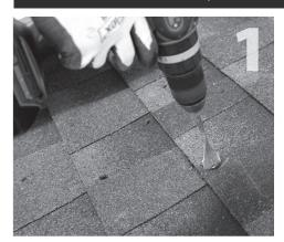
Mark center of rafter. Using the flashing as a template, mark the drill point so the flashing reaches up into the 3rd shingle course. Drill your conduit hole next to the rafter so you can secure the conduit below the roof surface (see Drawing 2). For 1/2" conduit, drill 7/8" hole; for 3/4" conduit, drill 1" hole; for 1" conduit, drill 1-1/4" hole.
