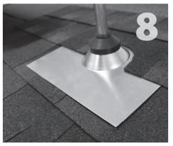
Slide collar over the conduit all the way down to the flashing.
