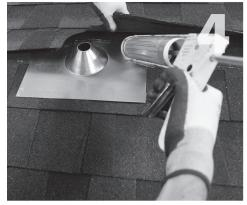
Slide flashing into place over drilled hole and apply a bead of sealant across the top side of the flashing under the 2nd shingle course. Be careful not to rip or tear shingles.
