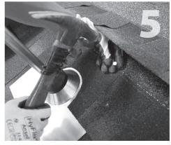
Under the 3rd course and through the 2nd course, secure flashing with 2 roofing nails at the top corners of the flashing at the nail line. Apply sealant over nail heads.
