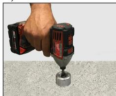
STEP 3: Using a cordless impact wrench, fasten lag bolt to rafter through base until seated.
