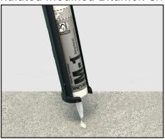
STEP 2: Apply a generous amount of roof sealant into pilot hole.
