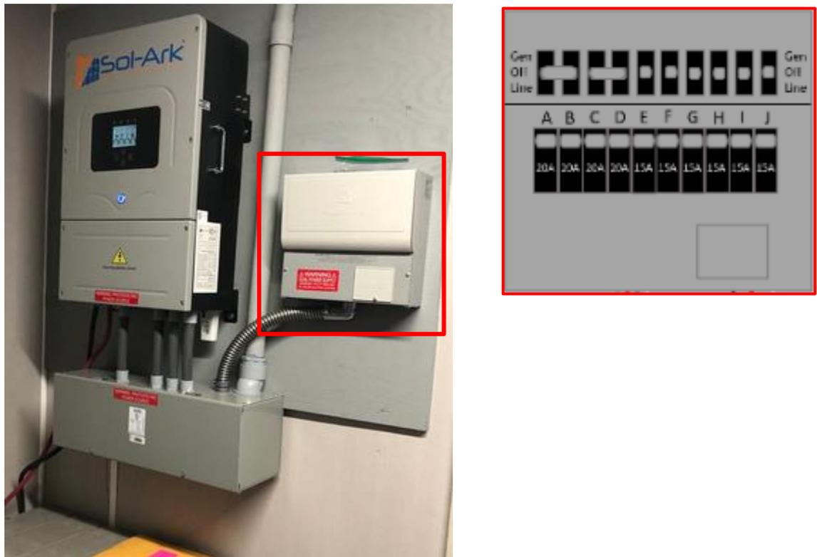
Figure 7.0 – Transfer Switch Kit
