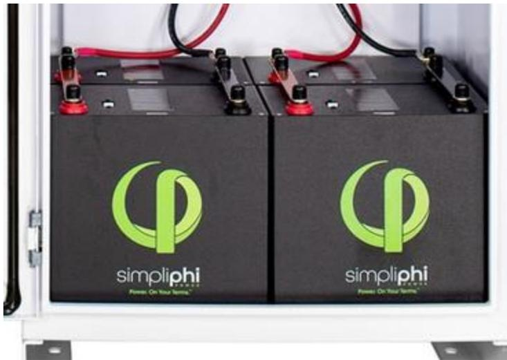
**Figure 9.0 – Interconnecting Busbars Parallel the Batteries in Sets of Two**
