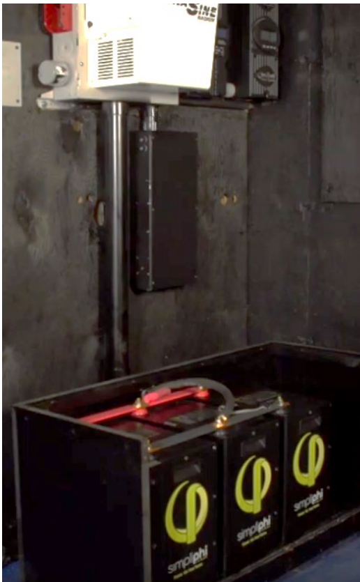
Figure 4.0 – Three PHI Batteries Paralleled Using Direct Bussing
