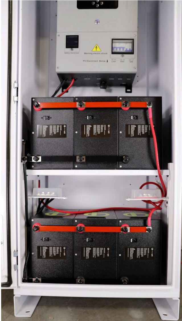
Figure 5.0 – Six Total PHI Batteries are Directly Bussed in Two Sets of Three, then Paralleled Using Cabling to a Single Positive Terminal Block and a Single Negative Terminal Block
