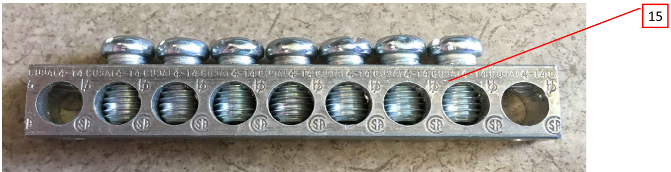
Photo 4 - Grounding Bar
