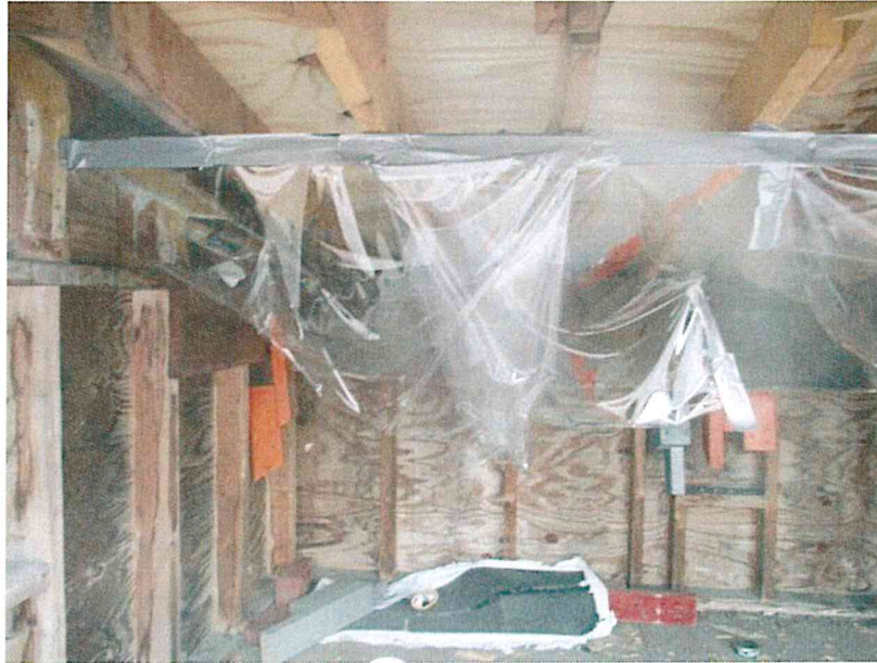
Photo No. 9 Underside of Test Specimens #1 and #2 After Testing
